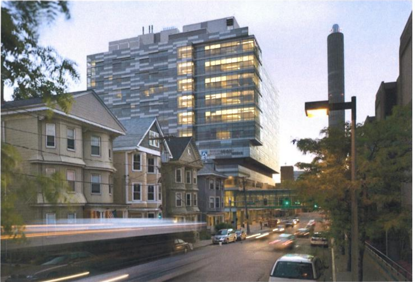
The Brigham and Women's Hospital Shapiro Center in Boston (©Anton Grassl/Esto)
