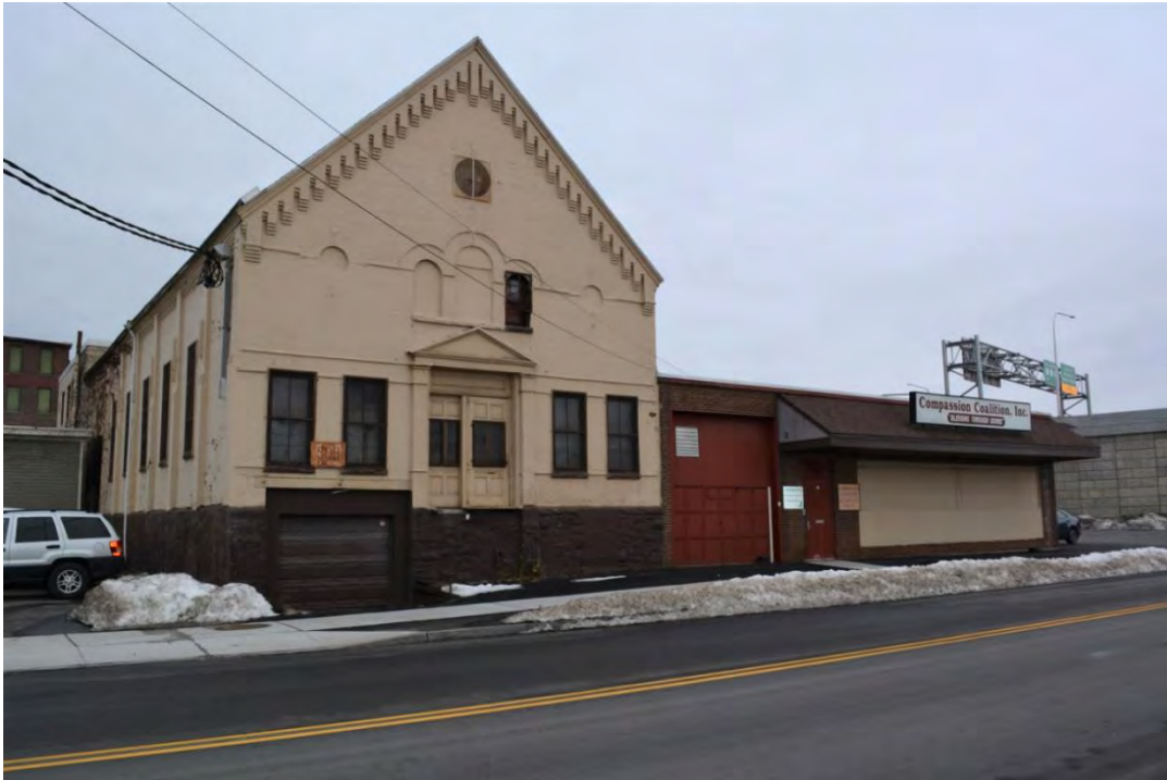
Photograph 3.6. Utica Turn Hall/Utica Turn Verein at 506 Columbia Street (shares address with 509 Lafayette Street), facing southwest (Panamerican 2018).
