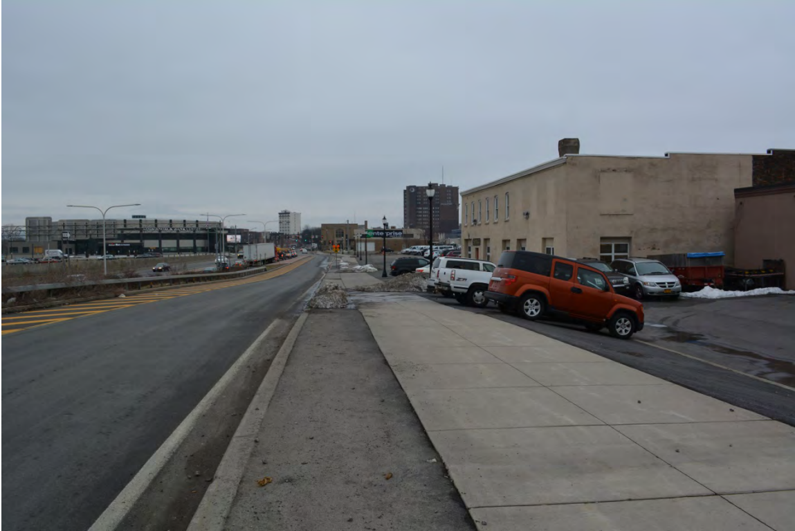
Photograph 5. Along Oriskany Street West from State Street, facing east (Panamerican 2018).
