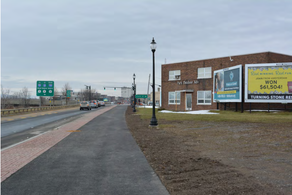
Photograph 1. Facing east on access road to Oriskany Street West from near northwest corner of the Project at State Route Highway 5 overpass (Panamerican 2018).
