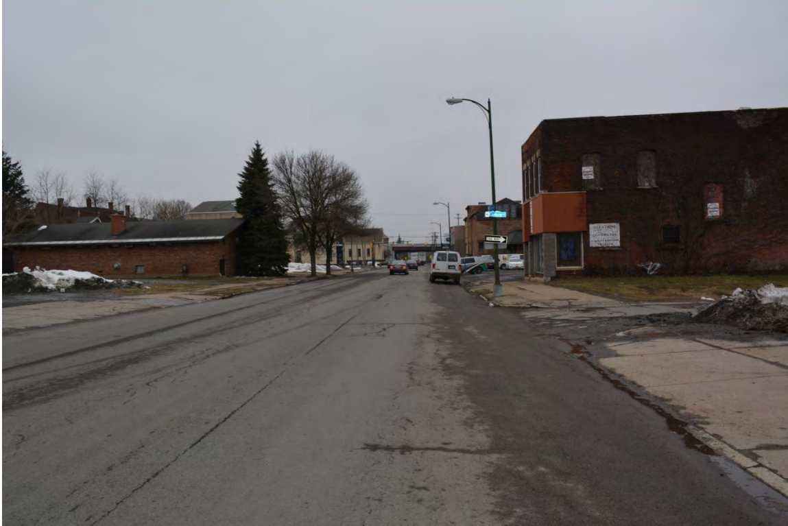
Photograph 13. Along Lafayette Street, toward Carton Avenue, at right, facing west (Panamerican 2018).
