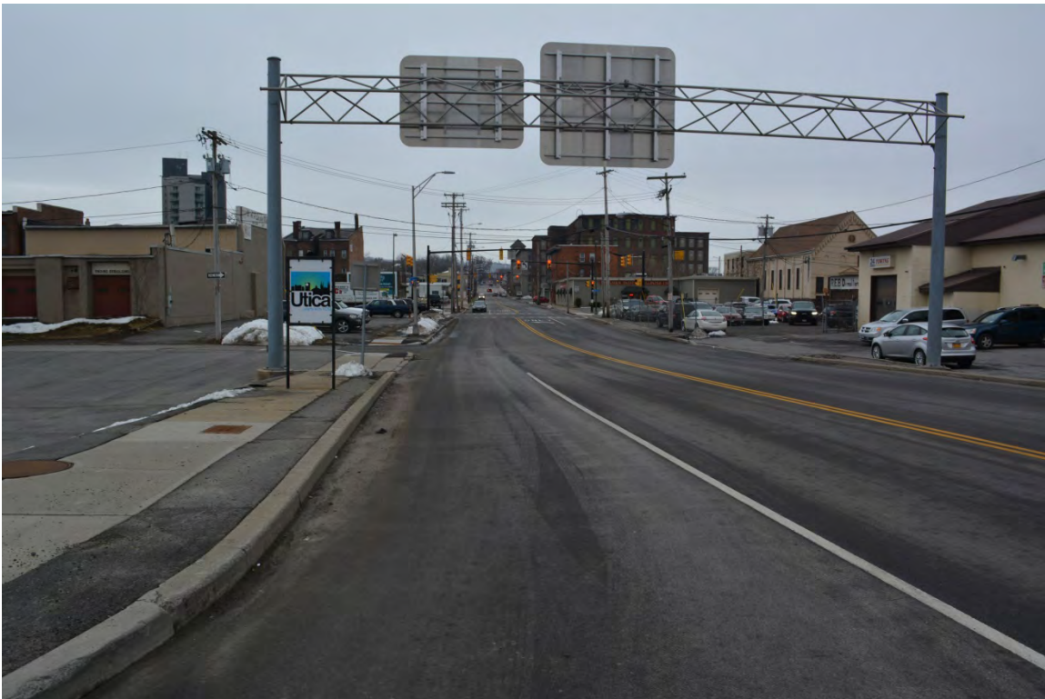
Photograph 4. Along State Street from Oriskany Street West, facing south (Panamerican 2018).
