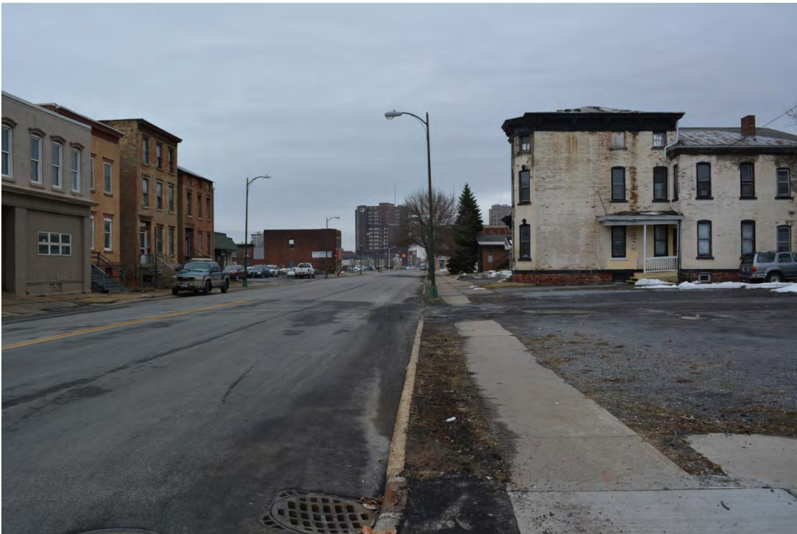
Photograph 20. Along Lafayette Street from State Street with the 440-444 block at left, facing west (Panamerican 2018).
