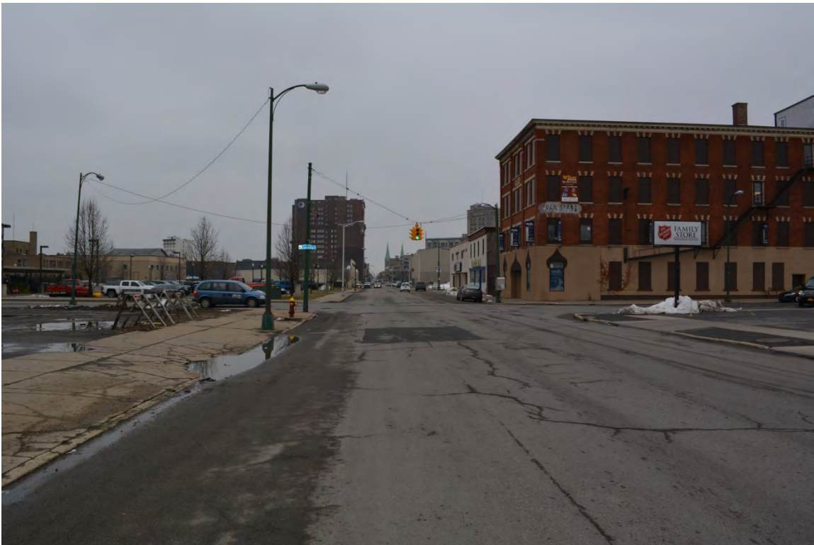
Photograph 12. Along Lafayette Street toward intersection with Cornelia Street, facing east ( Panamerican 2018 ).
