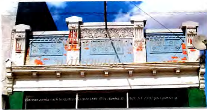
Terracotta cornice c. 1880- 430 Columbia St.
