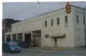
Interurban Trolley Garage- 300 Lafayette St.
