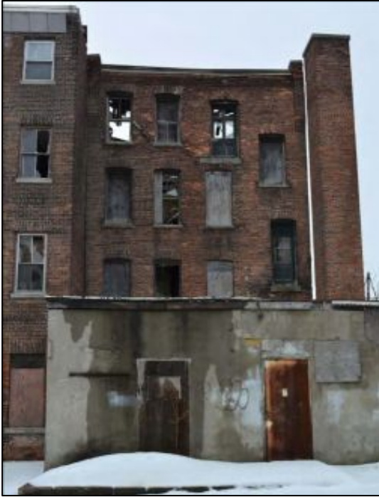
Figure 7. 336 Columbia Street Facing South
