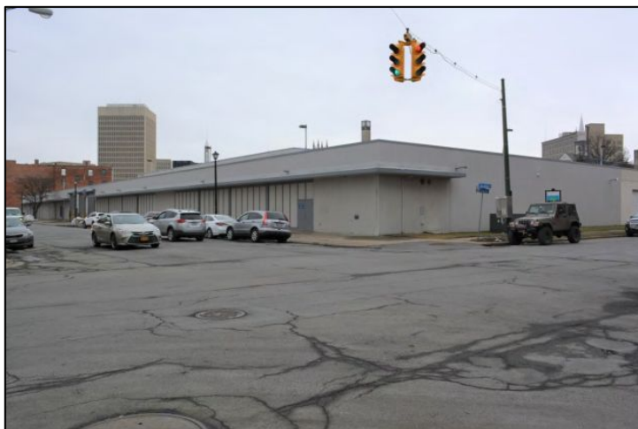
Figure 6. 335 Columbia Street Facing Southeast
