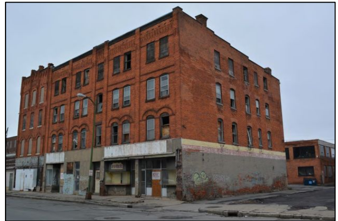
Figure 8. Haberer Building Looking Northwest (336 Columbia Street)
