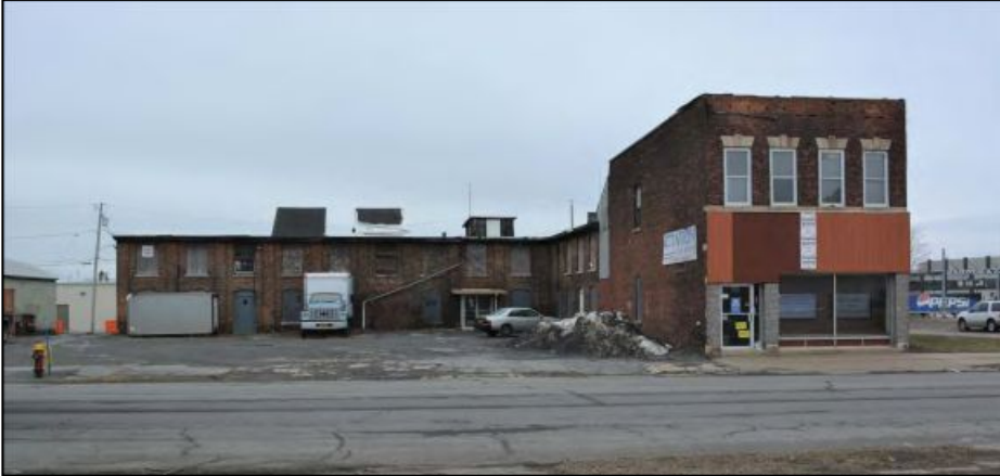
Figure 12. 418 Lafayette Street Facing North
