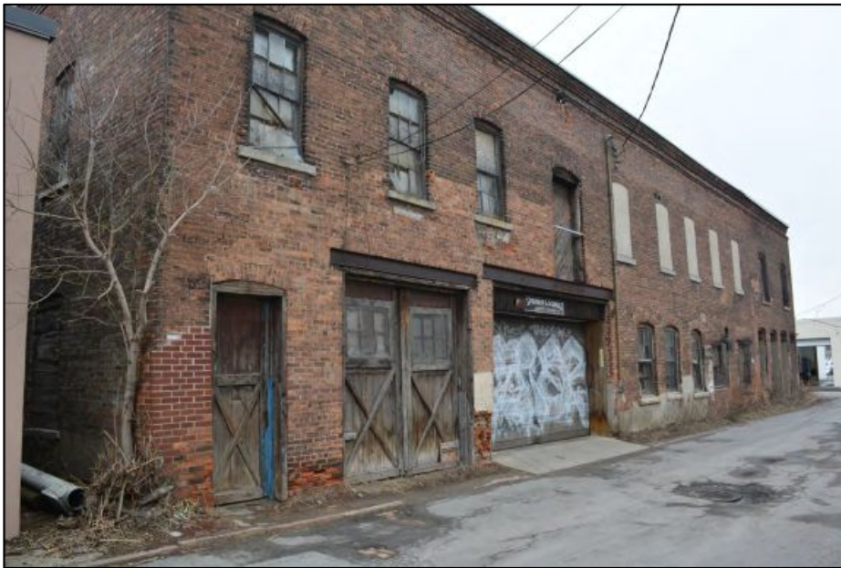
Figure 23. 529 Oriskany Street Looking Northeast
