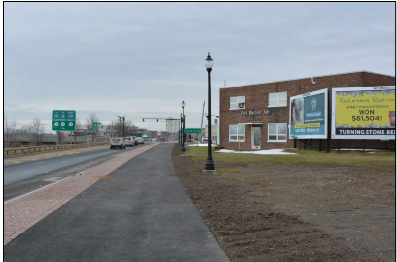
Figure 29. Existing Conditions: Oriskany Street from the Northwest.
