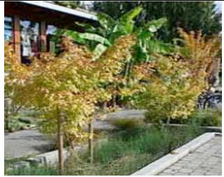
Also known as infiltration swales, biofilters, grassed swales, or in-line biorentention, bioswales are vegetated open channels specifically designed to attenuate and treat stormwater runoff for a defined water volume. Bioswales intentionally promote slowing, cleansing and infiltration along the way, thereby reducing runoff volumes into the Utica stormwater systems.
