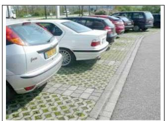
Permeable pavement can be used instead of standard asphalt and concrete for surfacing sidewalks, driveways, parking areas, and many types of road surfaces.
